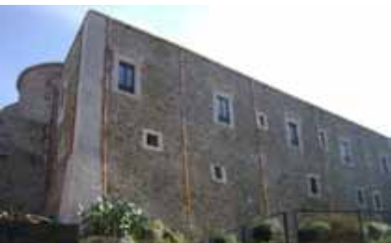
Sant'Agata di Militello: view of the west side of the castle seen from the Saracen Baglio and on the left the ancient access with two towers
